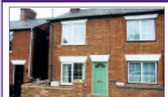
A refurbished two double bedroom end of terrace property close to local High Street. Unfurnished. Available now.
